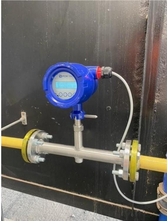
Figure 10: Fox Thermal Flow Meter behind kiln
