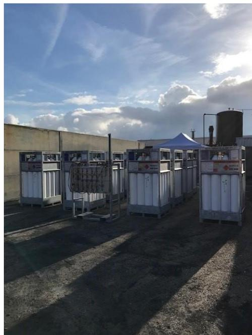
Figure 9: Hydrogen MCPs onsite
