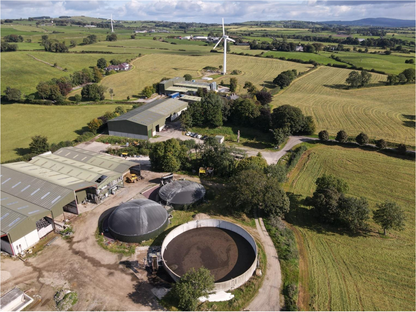
Figure 1- Aerial Picture of Hillside Combined Renewable System
