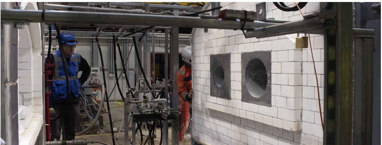
Figure 5: Combustion Test Bed Backwalls Used at the Glass Futures Facility
