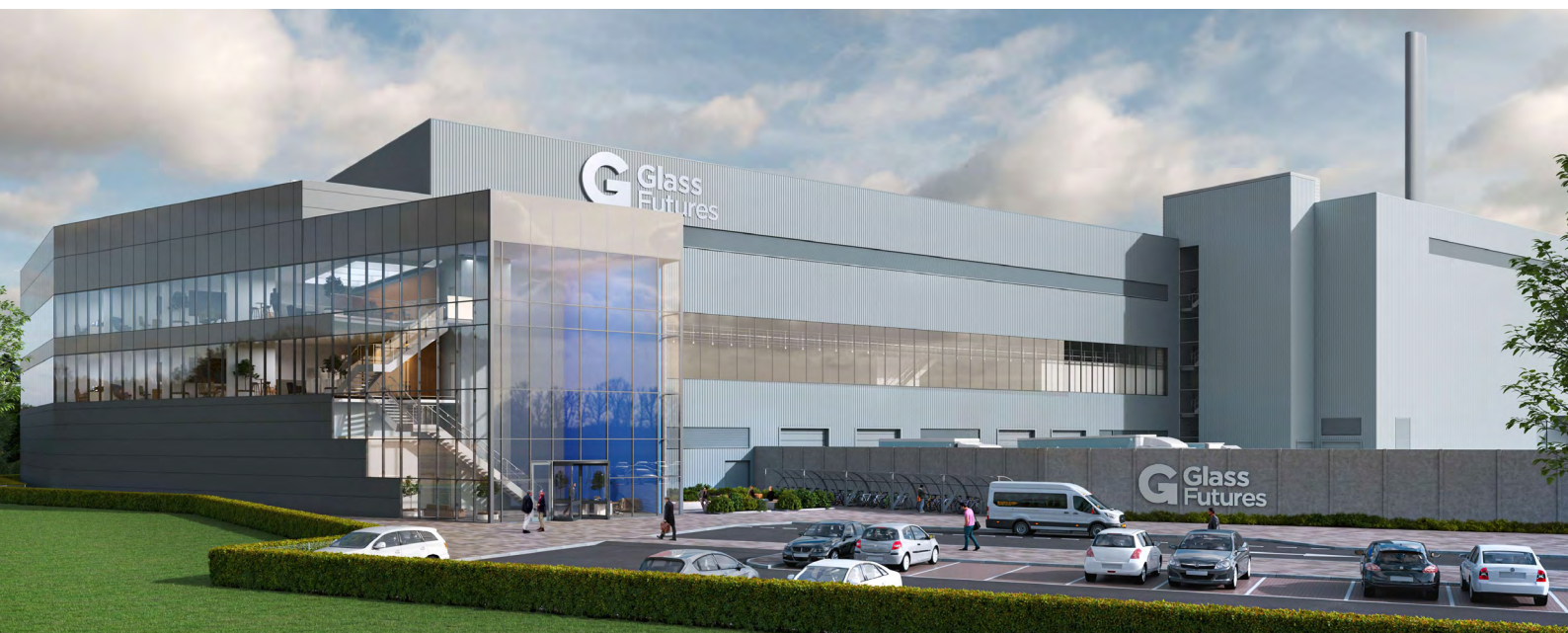
Figure 14: Glass Futures' Pilot-scale 30 t/day R&D Facility at St Helens
