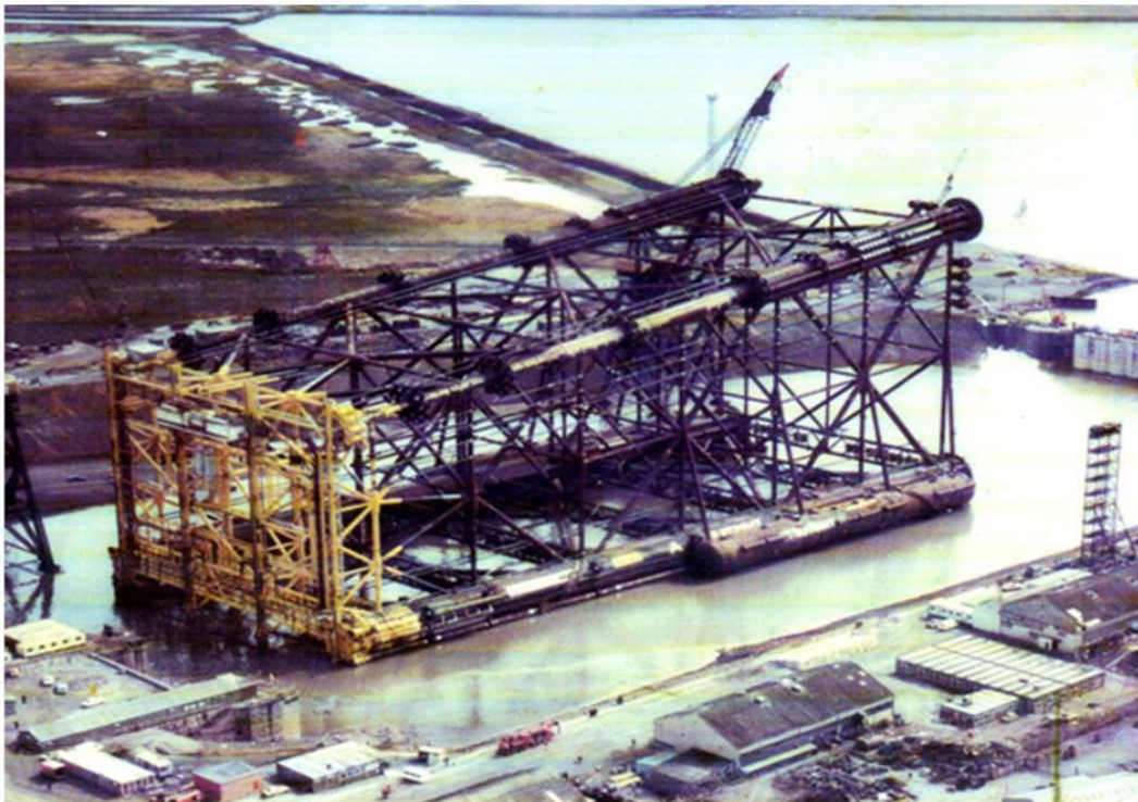
Figure 2.1.5: Thistle jacket fabricated at Greythorpe Dry Dock, Middlesbrough
