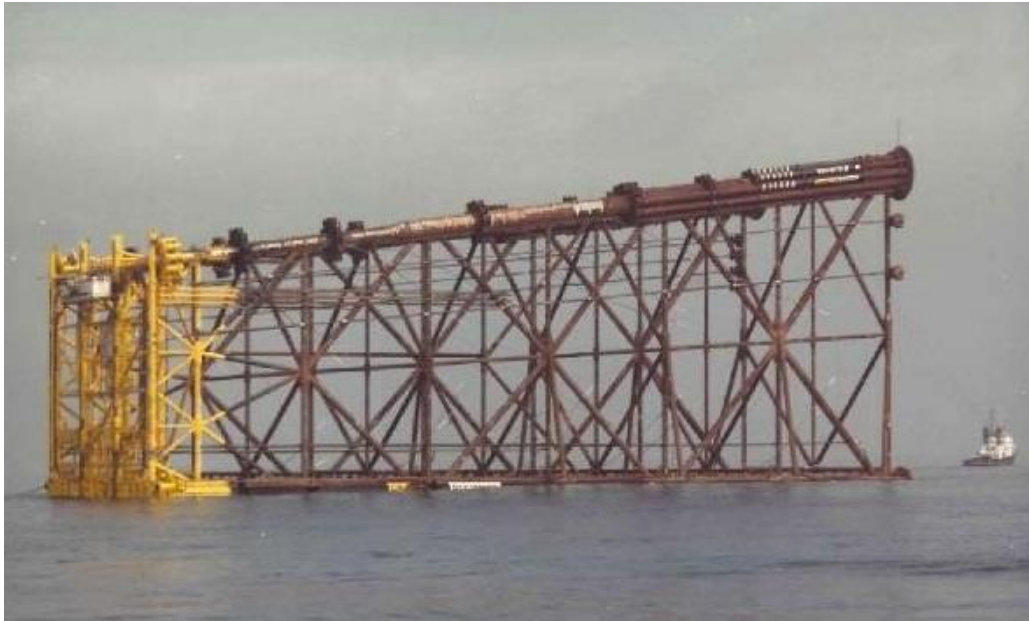
Figure 2.1.6: Thistle jacket immediately prior to upending
