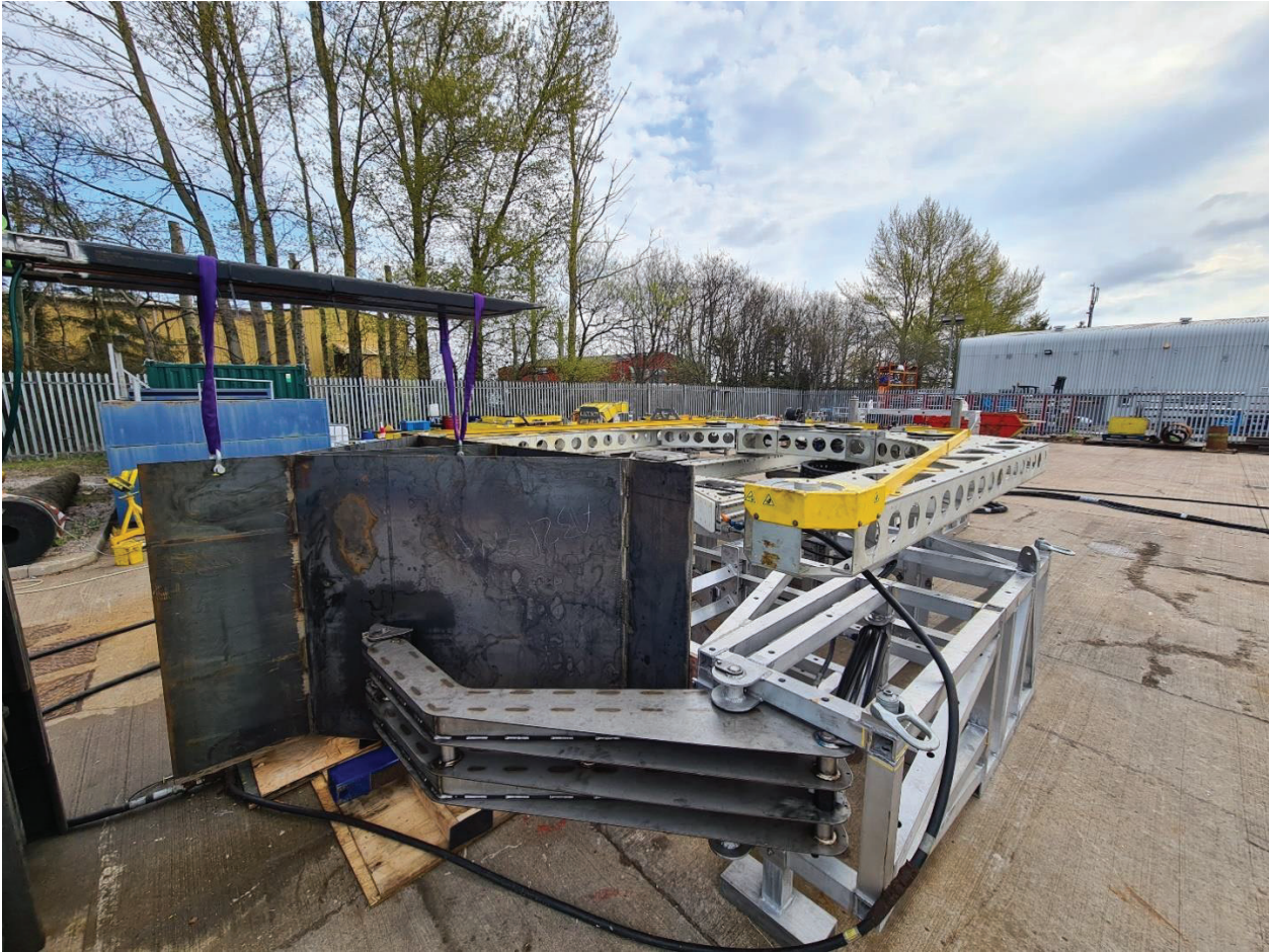
Figure 3-4: Anchortech pile with the 'Machtech TM ' 120" DWCM.
