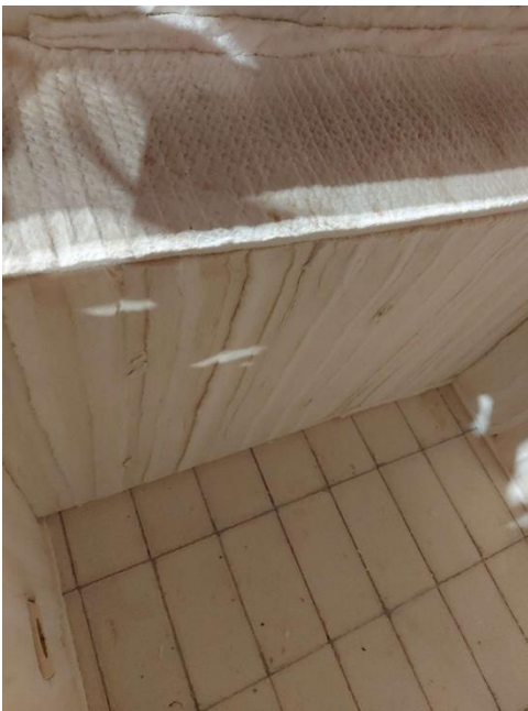
Area at side burner no damage viewed
