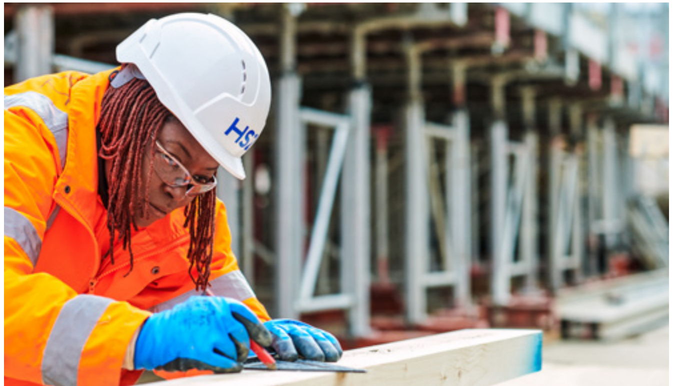
A worker at Old Oak Common station.
