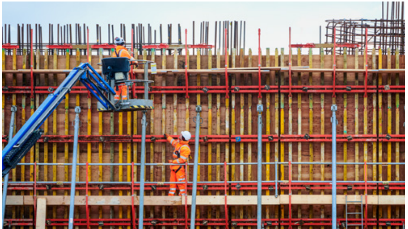
Working safely at height at the Kingsbury site.
