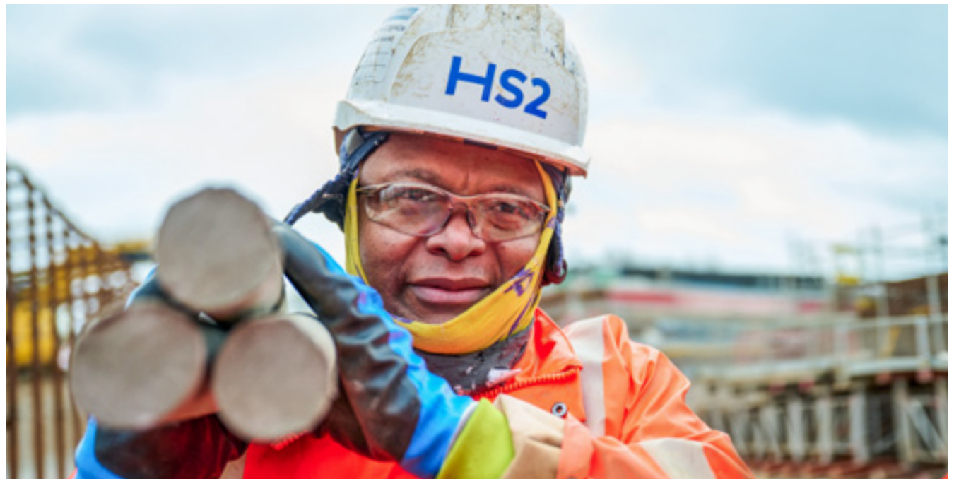
Construction worker at Old Oak Common station.
