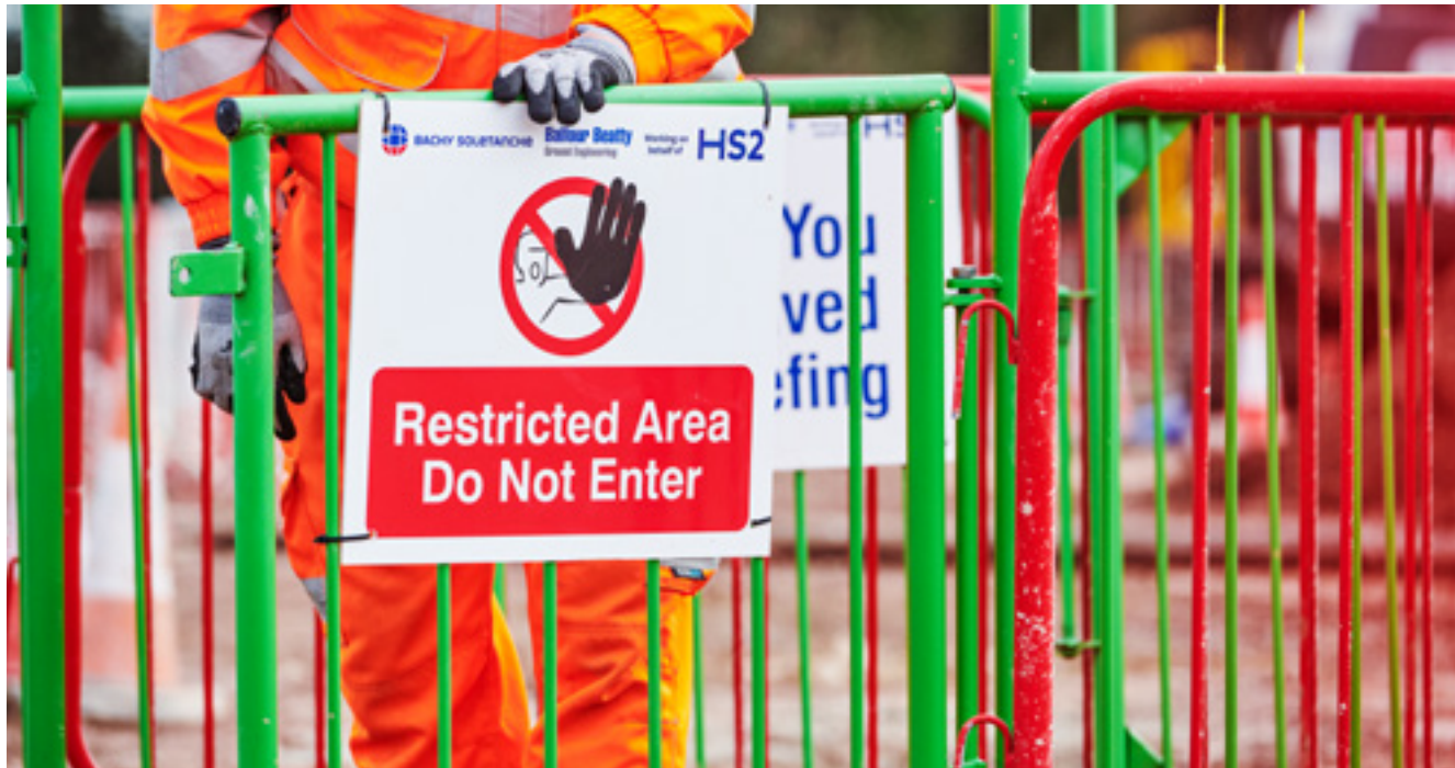
Security signs at HS2's site in Kingsbury, Warwickshire.
