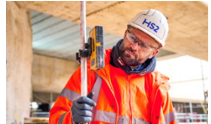
Measurements being taken at Old Oak Common station.
