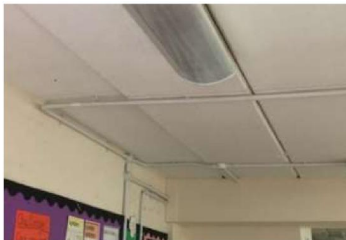
Figure 3 – Differential Deflection of Roof Planks
