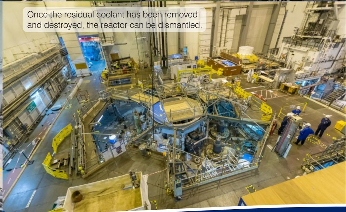
Once the residual coolant has been removed and destroyed, the reactor can be dismantled.
