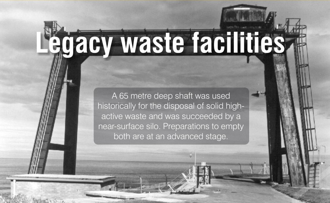
A 65 metre deep shaft was used historically for the disposal of solid high-active waste and was succeeded by a near-surface silo. Preparations to empty both are at an advanced stage.
