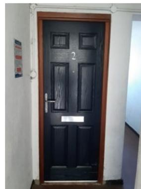
Composite flat entrance doors are a relatively modern innovation (dating from the 1980s onwards) and have become popular because of their attractive appearance and low maintenance. A typical composite door comprises a thin layer of glass reinforced plastic (GRP), or thermoplastic material, with a core (which can comprise various materials, such as phenolic foam) to provide the fire resistance. In older blocks of flats, they will be found only as replacements for original timber doors.
