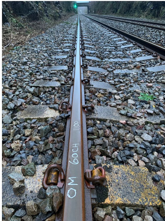
Figure 18: Railhead condition on the line between Lonlas Tunnel and Dynevor Junction (courtesy Network Rail).
