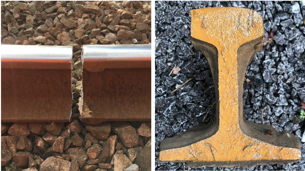
Figure 8: The rail break at Pencoed, in-situ (left-hand image) and its fracture face (right-hand image) (photos courtesy of Network Rail).
