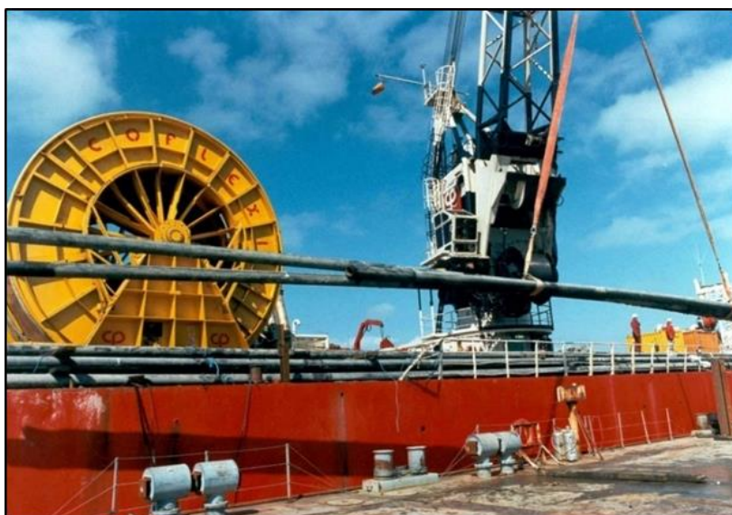
Figure 9: Pipeline Cut into Sections for Recovery
