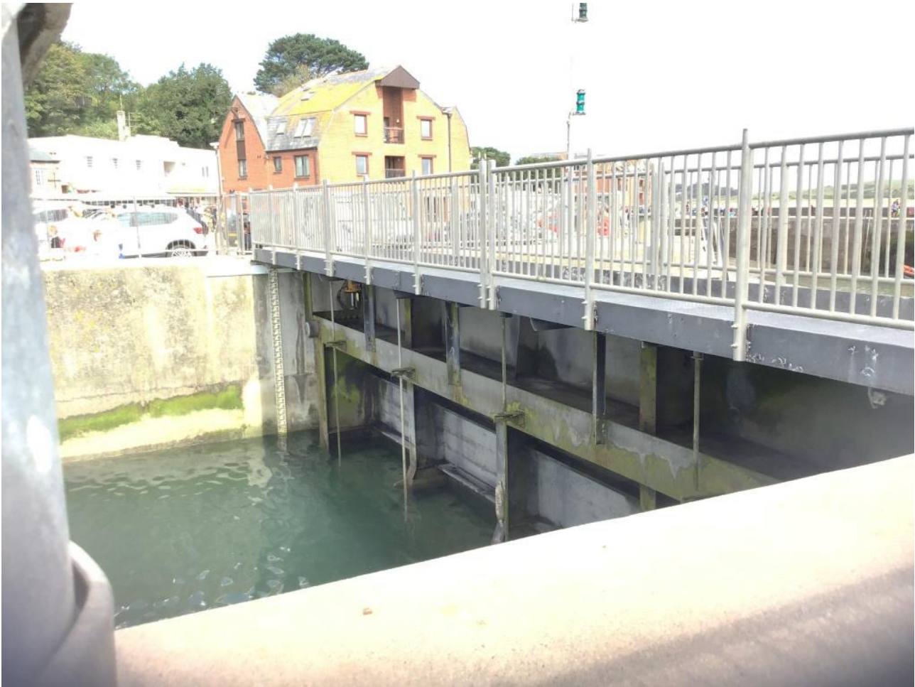
Figure 5: an image of the Padstow tide gate in operation and contractors during refurbishment project
