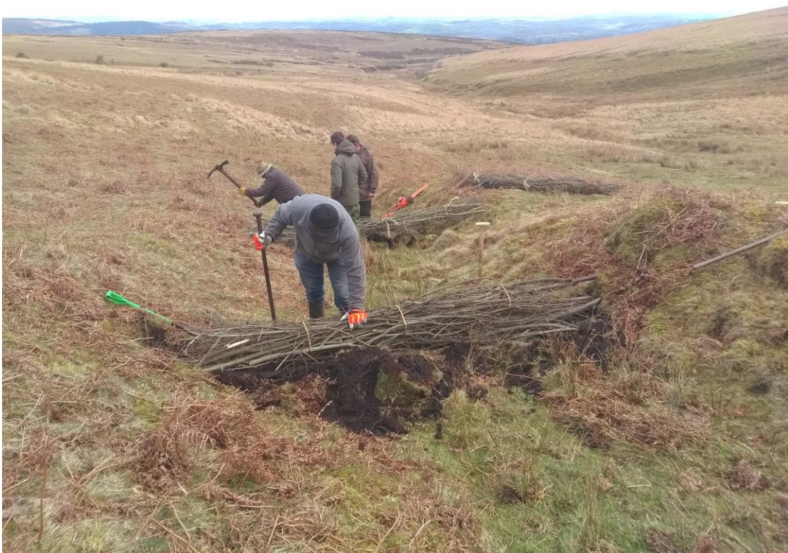
Figure 3: Dartmoor Commoners installing leaky dams in gulleys above Buckfastleigh, Devon
