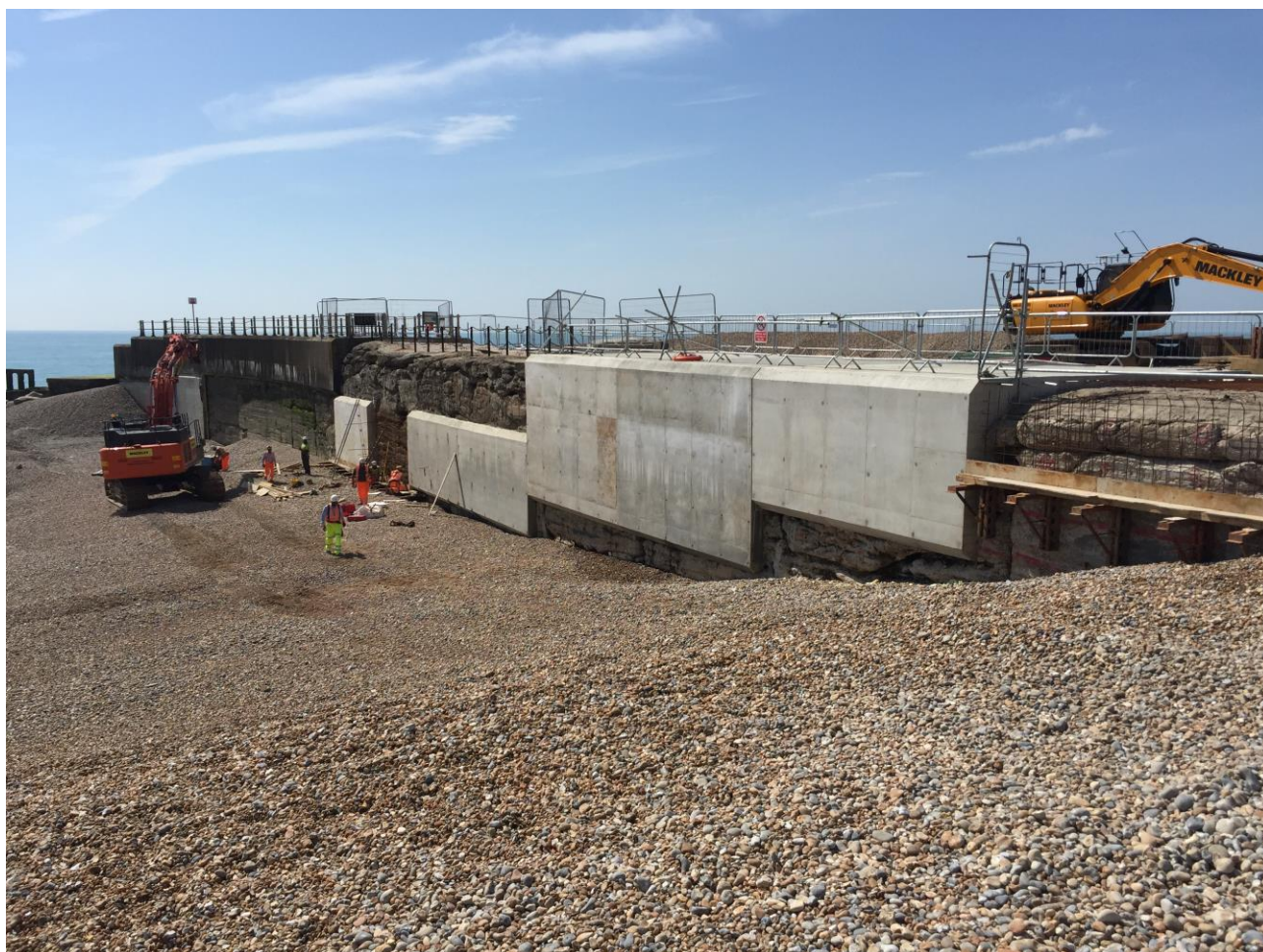
Figure 5: Hastings Coastal Defence Works, Stage 2
