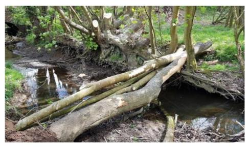
Figure 4: Leaky dam on River Bourne during installation in April 2019
