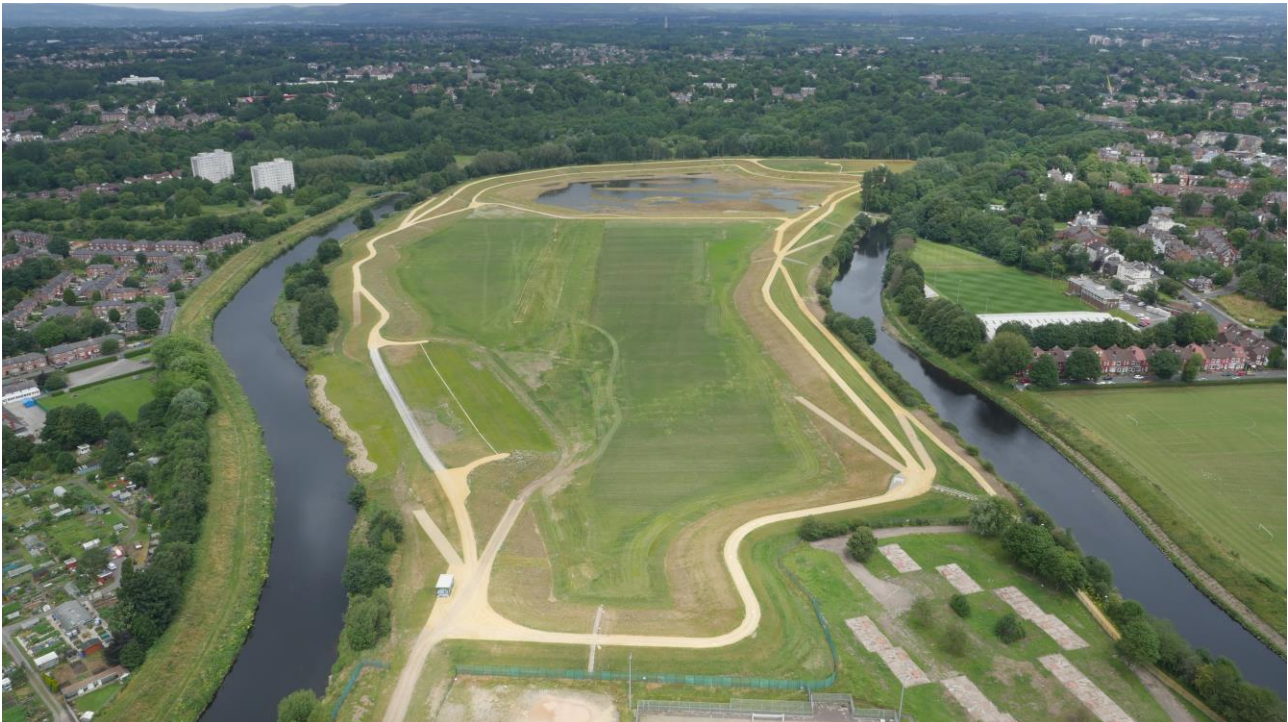
Figure 6: Aerial photo of Castle Irwell Flood Storage reservoir, Salford
