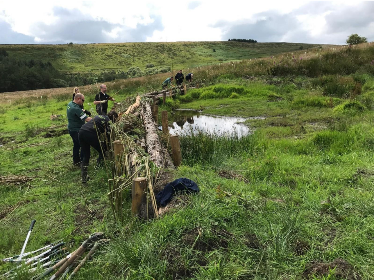
Figure 3: This image shows leaky woody barriers upstream Woodlands Trust, Smithills Estate NFM project. Live, of Bolton. Sep 2019.
