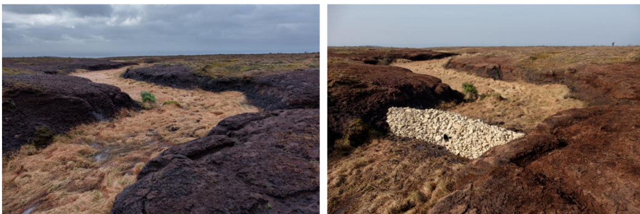
Figure 5: Stone Dam NFM interventions - before (left) and after (right)
