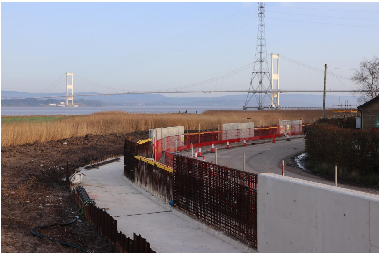
Figure 3: construction of the ASEA project
