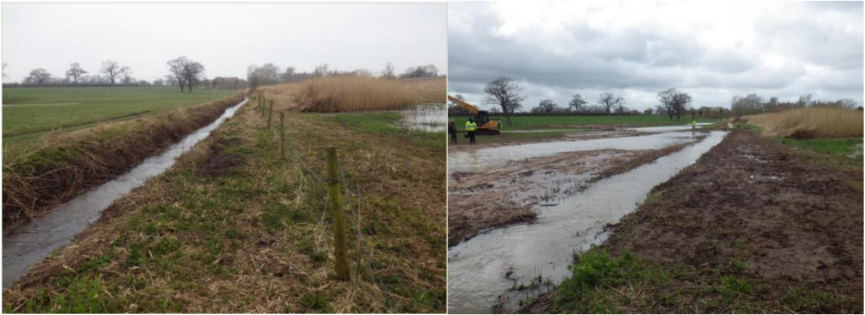
Figure 3: Mill Brook, Tattenhall before (left) and after construction (right)
