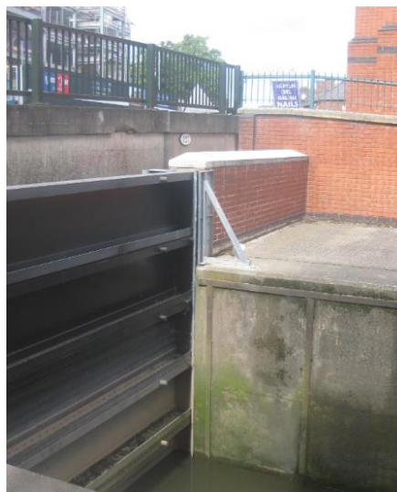
Figure 4: Demountable flood barrier at Dee Locks, Chester
