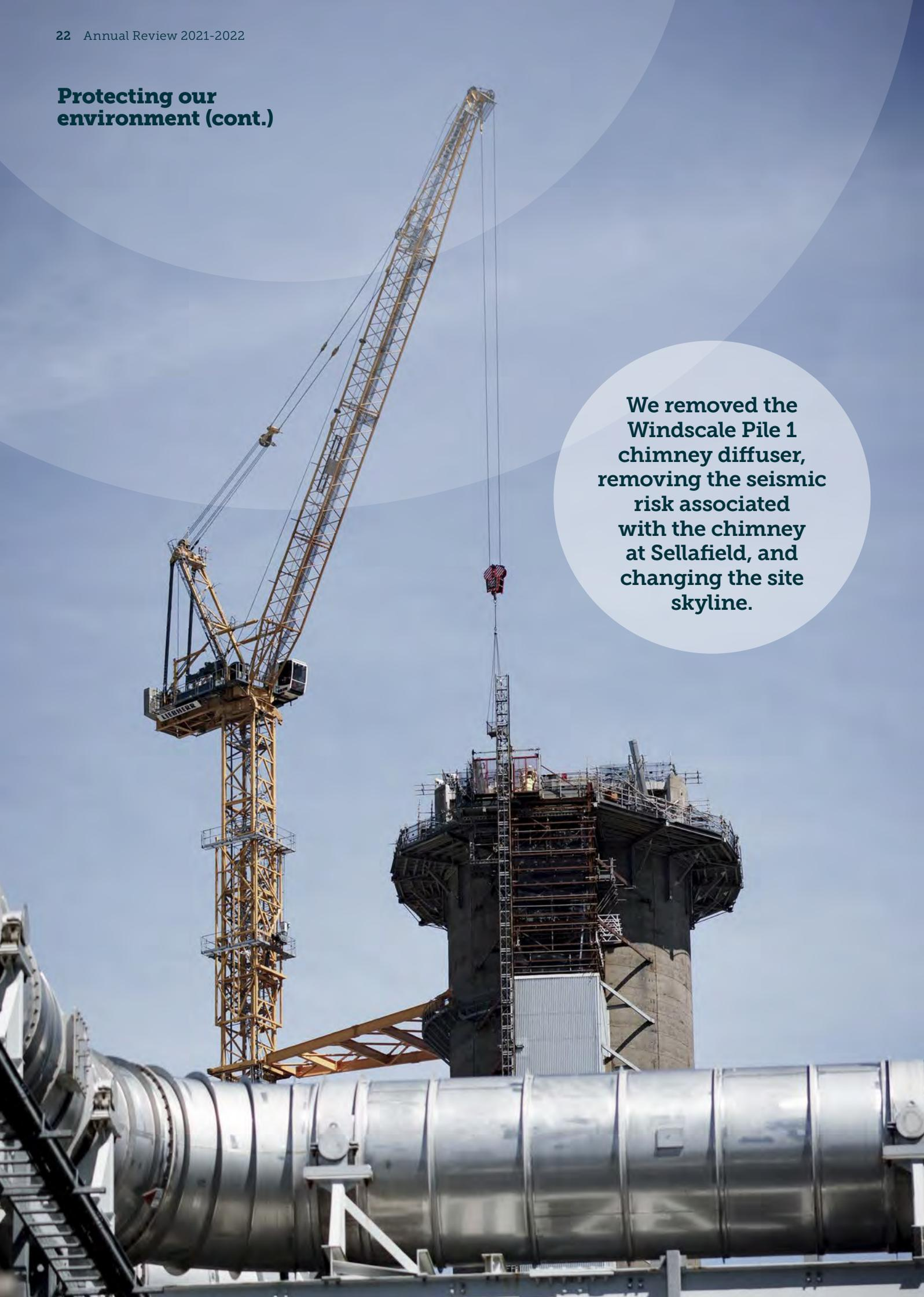
We removed the Windscale Pile 1 chimney diffuser, removing the seismic risk associated with the chimney at Sellafield, and changing the site skyline.
