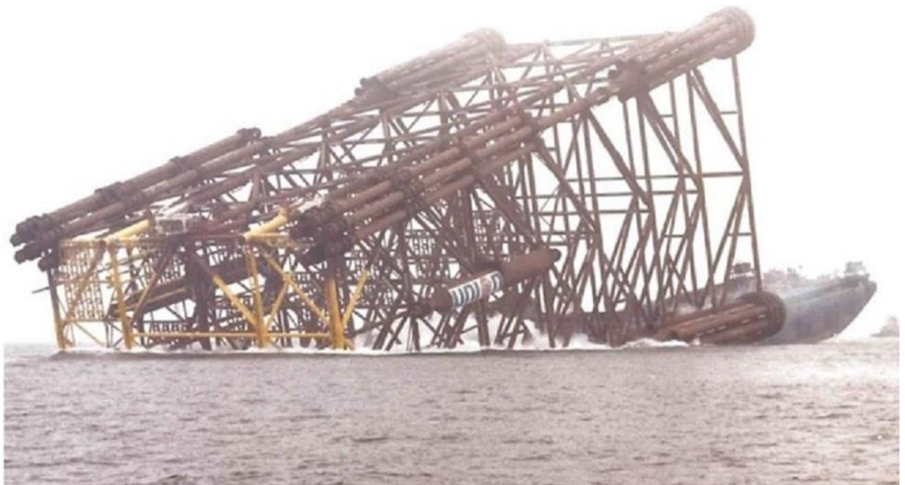
Figure 2.1.3: Heather jacket launch from McDermott Intermac 600
