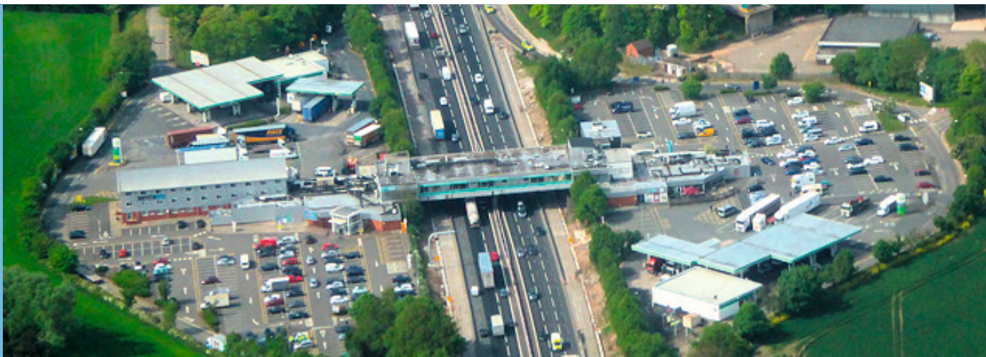
Knutsford motorway services and compound, Source: Motorway Services Online, Credit: David Dixon
