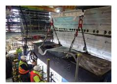
In the Magnox Swarf Storage Silo we made progress with the installation of the second Silo Emptying Plant and moved the first machine into position ready to start retrieving the waste held inside the silo.
