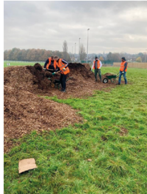
Project: May and Baker project Supporting with the ground levelling of the communal sports ground.
