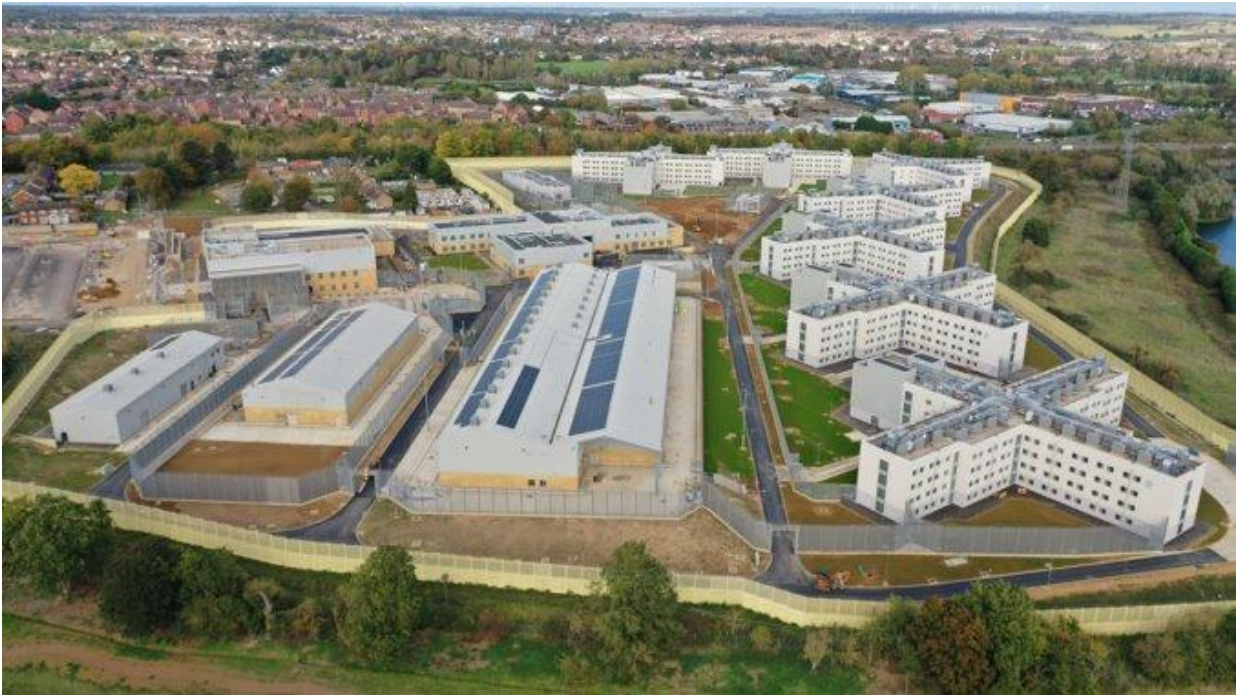
Image 1: HMP Five Wells, Wellingborough
