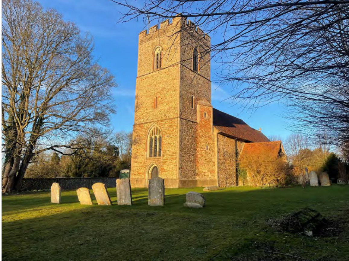
1. St Mary's Church, looking north-northeast
