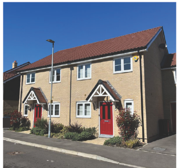
Fig 2.4.16 Buff Brick with Pitched Roof Porch
