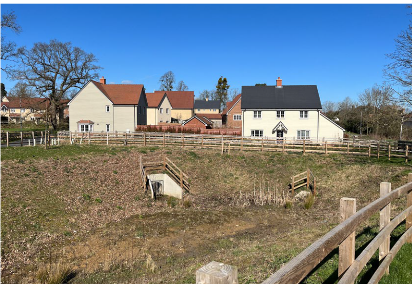
Fig 2.4.24 Naturalistic Drainage Basin
