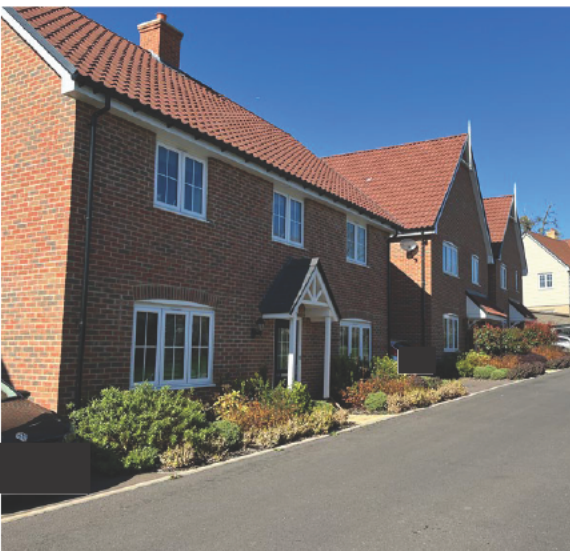
Fig 2.4.14 Red Brick With Pantile Roof
