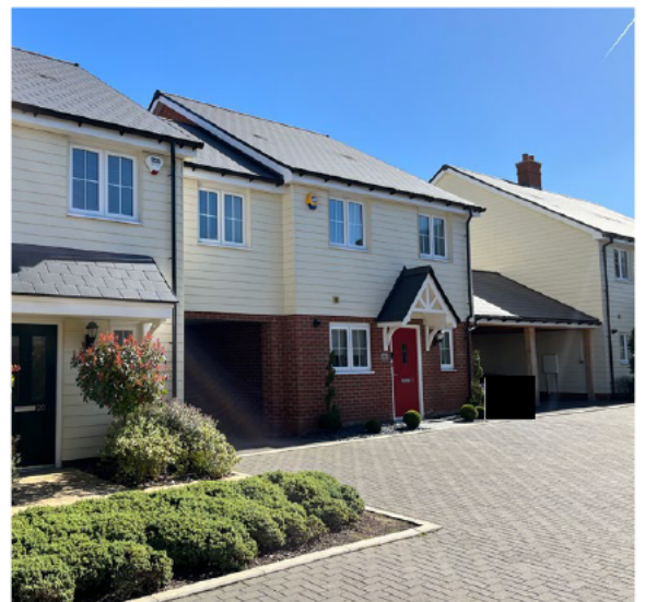
Fig 2.4.8 Shared Surface Courtyard
