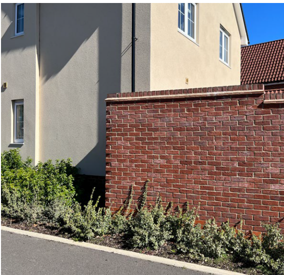
Fig 2.4.21 Brick Walls Facing Public Realm Areas
