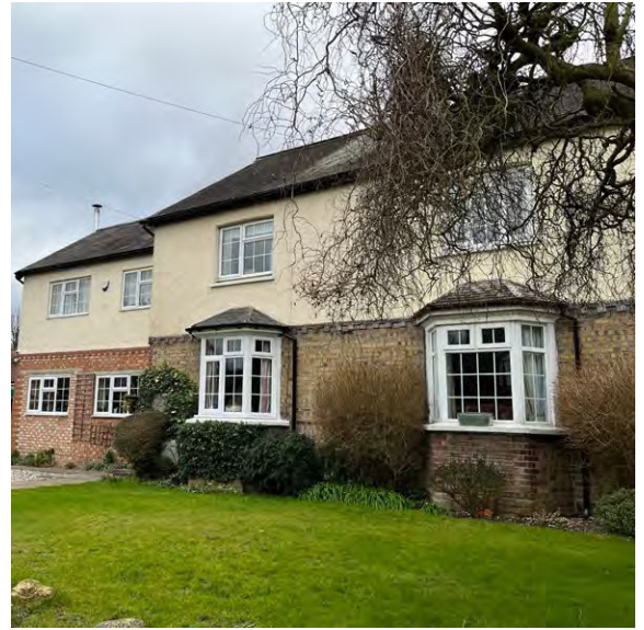
Fig 1.13.5 House along Park Road
