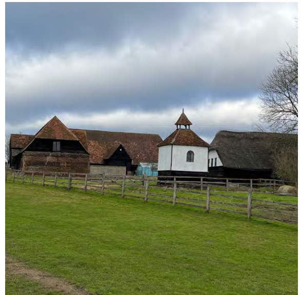
Fig 1.6.2 The Barns and Dovecote
