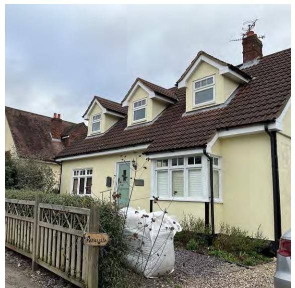
Fig 1.13.7 House along Park Road
