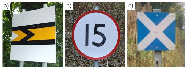
Figure 8: Photographs showing examples of a) a fixed distant signal, b) a 15 mph permanent speed restriction sign and c) an AWS cancel sign
