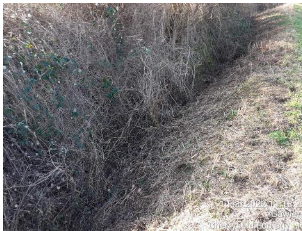
Figure 12a: Example of dry ditch (2022).
