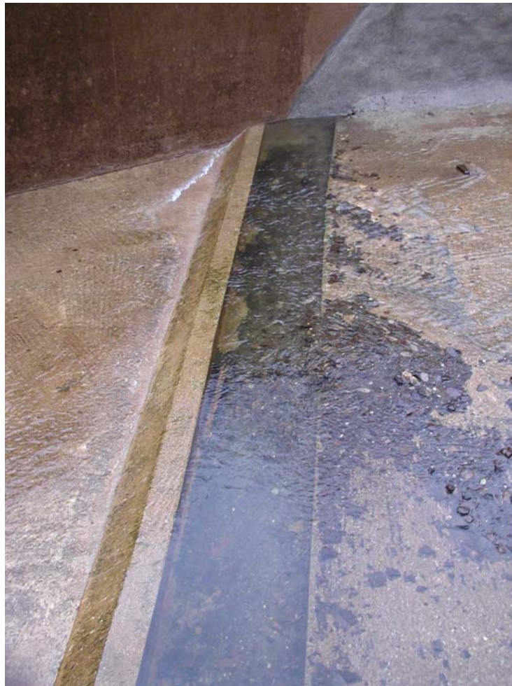
Figure 7.3: The eel bypass trough at the Backbarrow hydropower scheme on the River Leven, Cumbria (Spiby, 2004). The trough is formed along a diagonal in the floor of the headrace canal, with a submerged bywash at its downstream end. The flow in this picture is from right to left.
