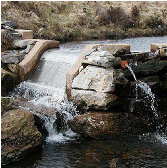
Figure 4.6: Example of a Screen B Coanda installation (Dulas Hydro).
