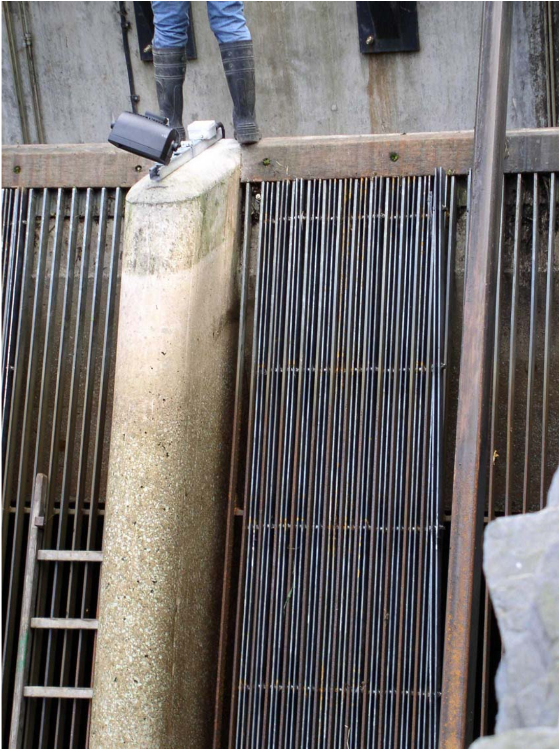
Figure 4.3: Vertical bar racks being overlaid with additional bars to reduce the effective bar spacing. The photograph was taken at the Backbarrow hydropower scheme in Cumbria during the process of adding bars and is incomplete as shown. The overlay screens only remain in place during the autumn eel migration season.
