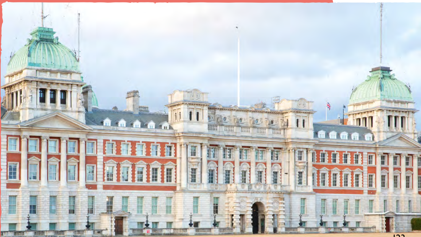
Image: The Department for Business and Trade headquarters at Old Admiralty Building
