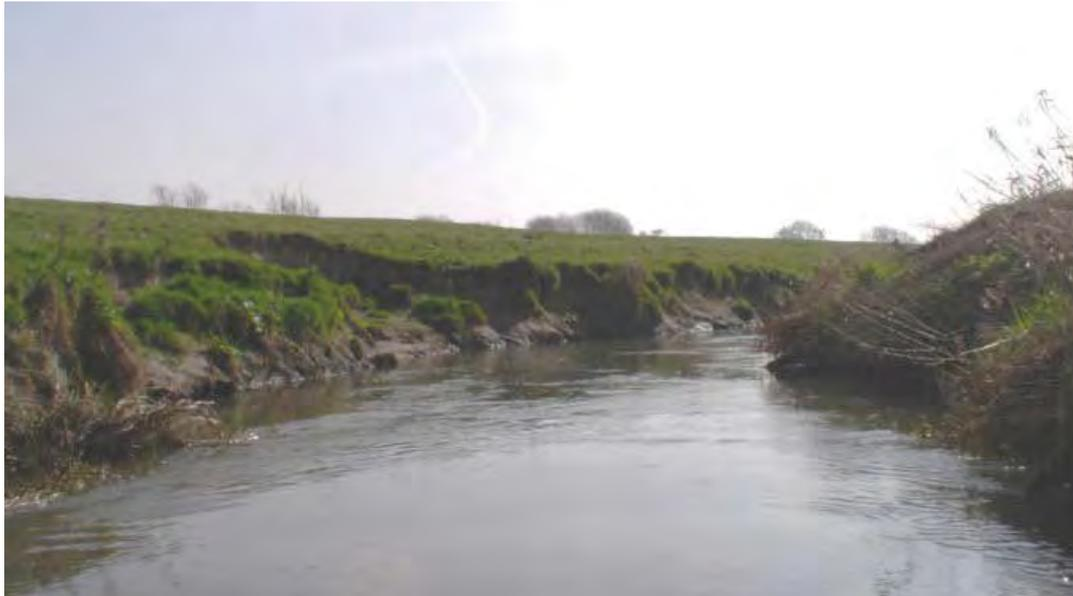
In this example, the river has had both banks and channel resectioned in the past. The channel is still clearly over-deepened and realigned, but the banks are beginning to naturalise in places (note lots of erosion, slumping and diversity in the bank profile on the left).
