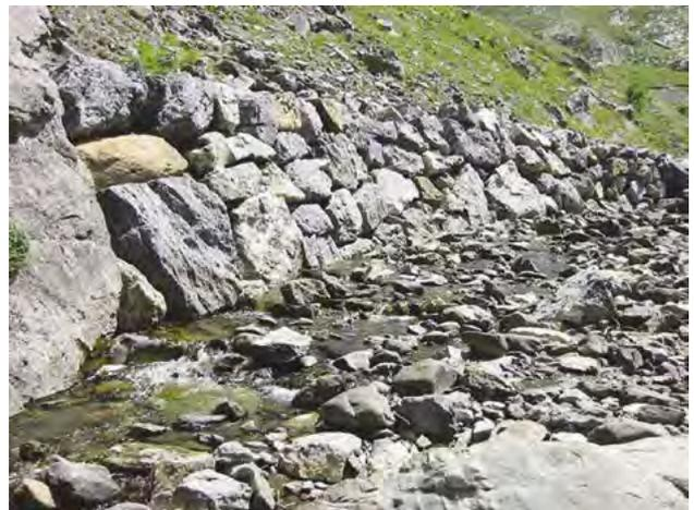
E1Ma Rip-rap bank material; placed (but not cmented), non-regular, blocks. Bank vegetation structure is recorded as bare.
