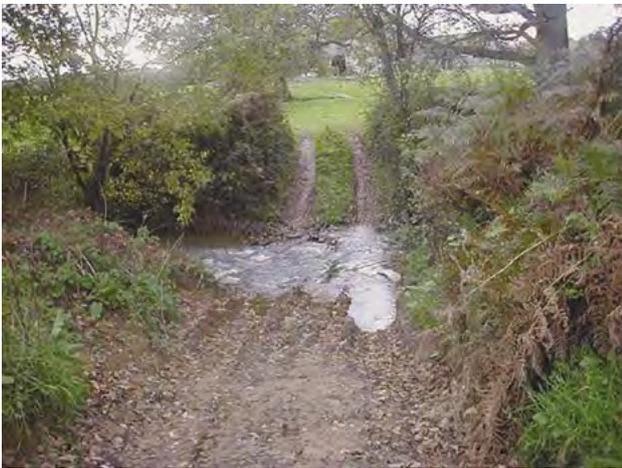
D5c Minor ford – farm track where bed and banks are of both composed of natural material, and there is no significant ponding impact from the ford.
