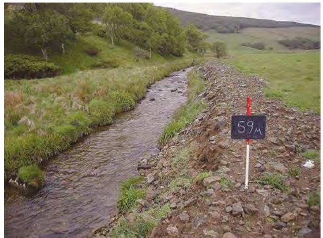
E6f Resectioned channel – this shows a mobile, gravel-bed, river that has been resectioned, with tell-tale spoil on the right.
