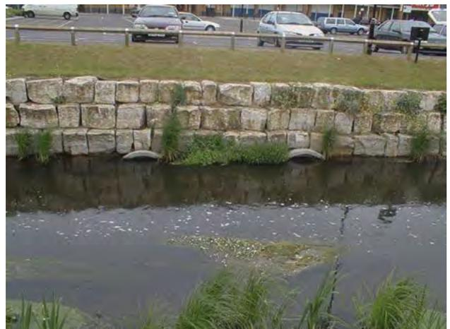
E1Mb Rip-rap bank material; placed (but not cmented), square, blocks. Note under-water 'pipes' for fish shelter (note in Section P).
