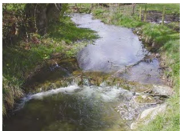
D1f Intermediate weir – wooden log construction, and water can leak through gaps.
