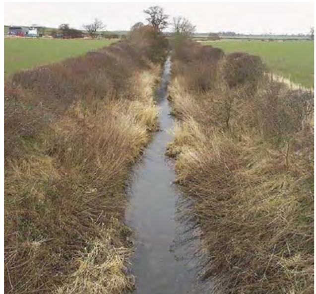
D7a An obviously realigned and over-deepened channel. Note hedge at the top of the bank that should be recorded as complex banktop vegetation structure.
