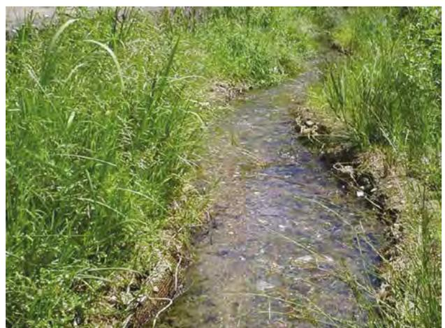
E1Pe Bio-engineering bank materials – here biodegradable hessian has been used in combination with reed planting and other vegetation.
