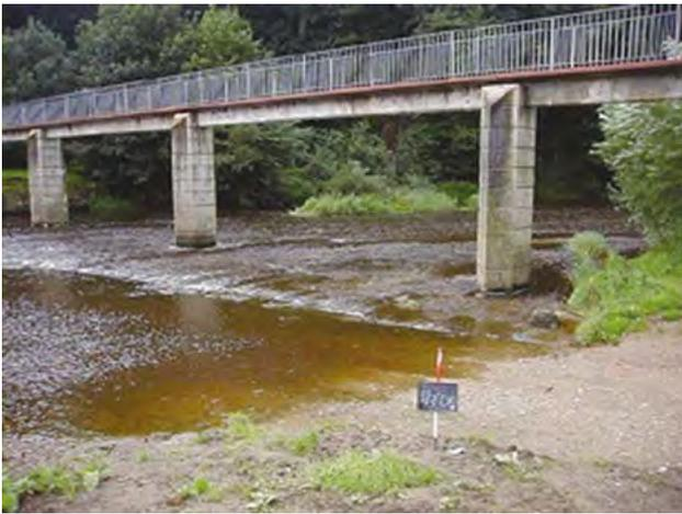
D5b Major ford – note the bed is composed of artificial material, but the banks are 'natural' gravel. Note major bridge downstream with in-channel supports.
