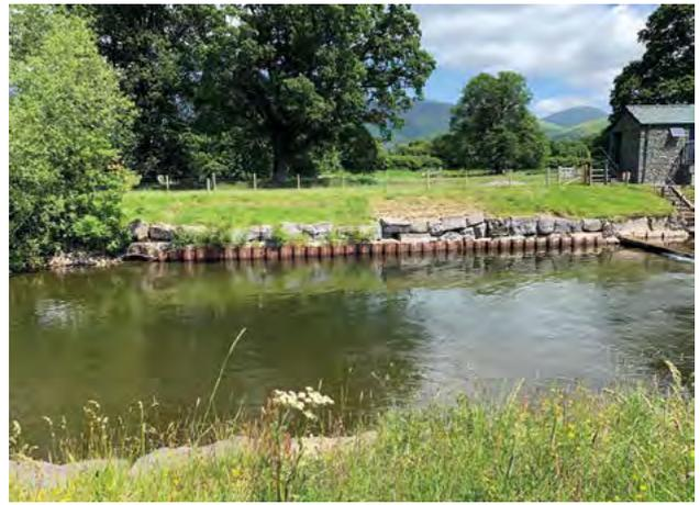
16b Reinforced bank – toe only; reinforcement is metal sheet piling and rip rap above. Note also bank is resectioned.
