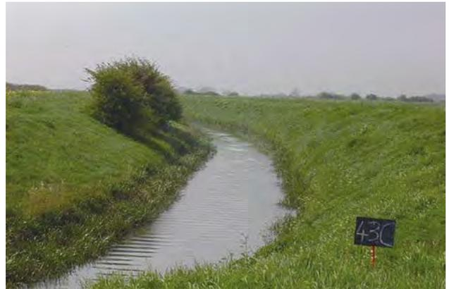
E6e Resectioned bank – this example shows river with few trees, very even gradients to the banks, and with the banktop width <4 times the banktop height indicating both deepening and resectioning.
