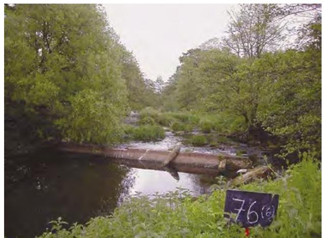
D6b This collapsed weir is recorded as a major deflector as it extends >20% across the channel.
