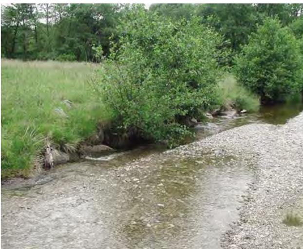
16a Reinforced bank – toe only; reinforcement is with large boulders (rip-rap). See also E1Ja,b, E1Ka, E1Oa.
