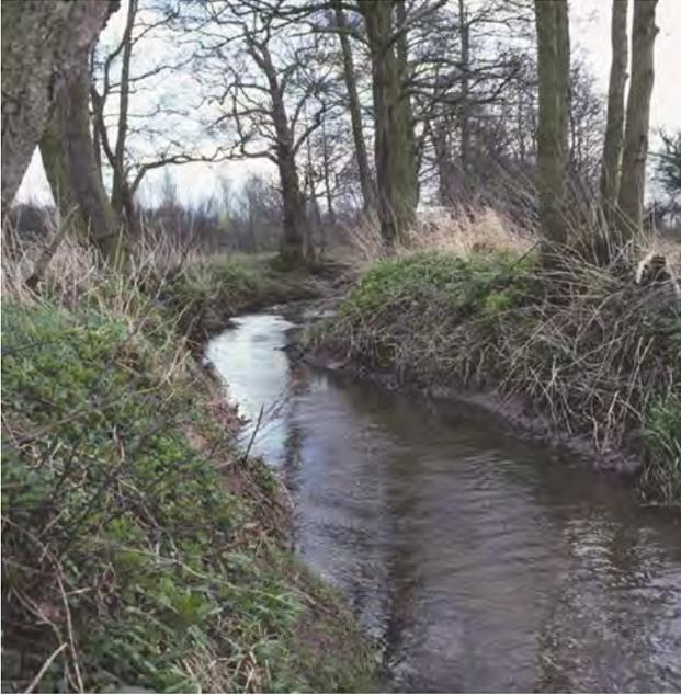
E6a Resectioned channel – typical signs seen here include deep channel *cf.* width, steep smooth-sloped banks, and even-aged trees only on top of bank. See also A1a-c, D8a.
