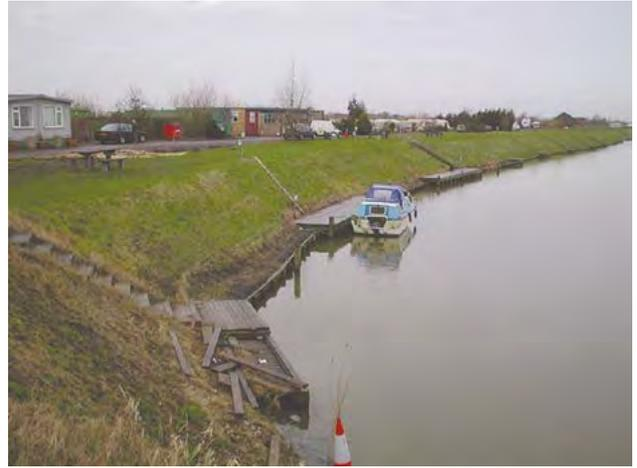
D6f Other artificial features – boat moorings. These extend 10-25m along the bank, so are classed as 'intermediate'.
