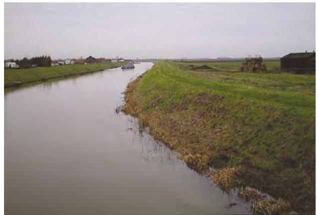
E2Da Embanked – note the earth embankment is placed on top of the natural bank (cf. set-back embankment, Section I).
