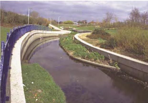
E2Cb Artificial Berm – formed by infilling wide, totally artificial, channel (here on both sides) to form a two-stage channel.
