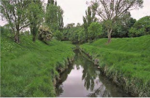
E2Ca Artificial Berm – formed by excavating bank material (here on both sides) to form a two-stage channel. Both the flat base of the berm, and the face of the top of the bank, constitute ‘bankface’. See also E1Hb, F18b.
