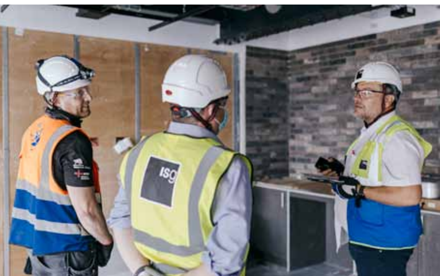
Birmingham, 23 Stephenson Street during construction
