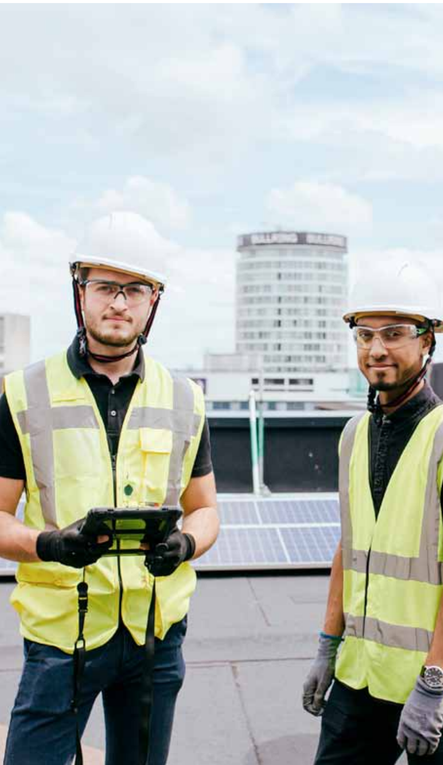
Solar panels installed at Birmingham, 23 Stephenson Street
