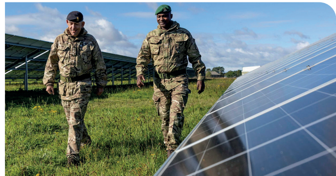
Army's first solar farm at the Defence School of Transport (DST) in Leconfield, East Yorkshire
