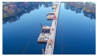
Four jetties have been built to support construction of the Colne Valley viaduct.
