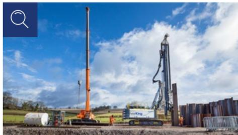
Sheet piling being installed for the Wendover Dean viaduct.
