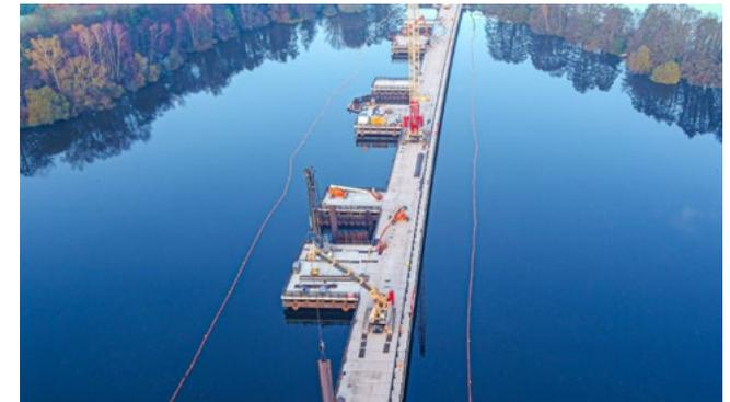
Four jetties have been built to support construction of the Colne Valley viaduct.
