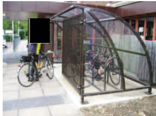
Covered shelter secured with lockable gates
