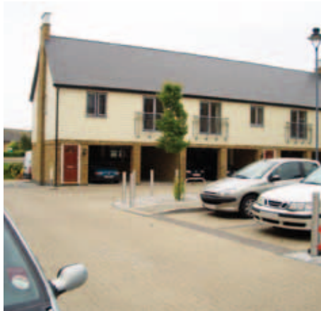
Undercroft parking facing onto central parking court
