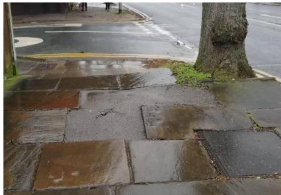
Uneven footway/pavement
