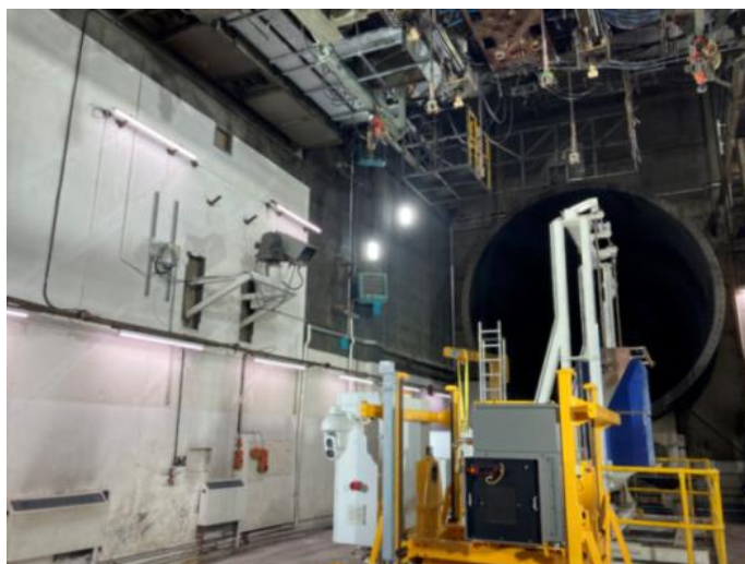
Figure 3: Rolls-Royce Test Bed 52, the demonstrator test location
