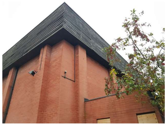
Photo 4. South-western elevation of B21 (Sports Hall).
