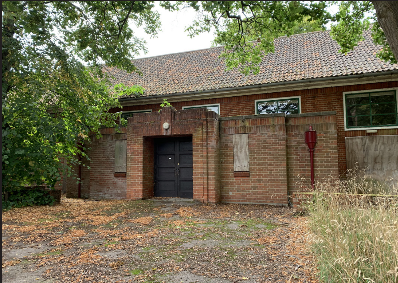
Assembly Hall entrance
