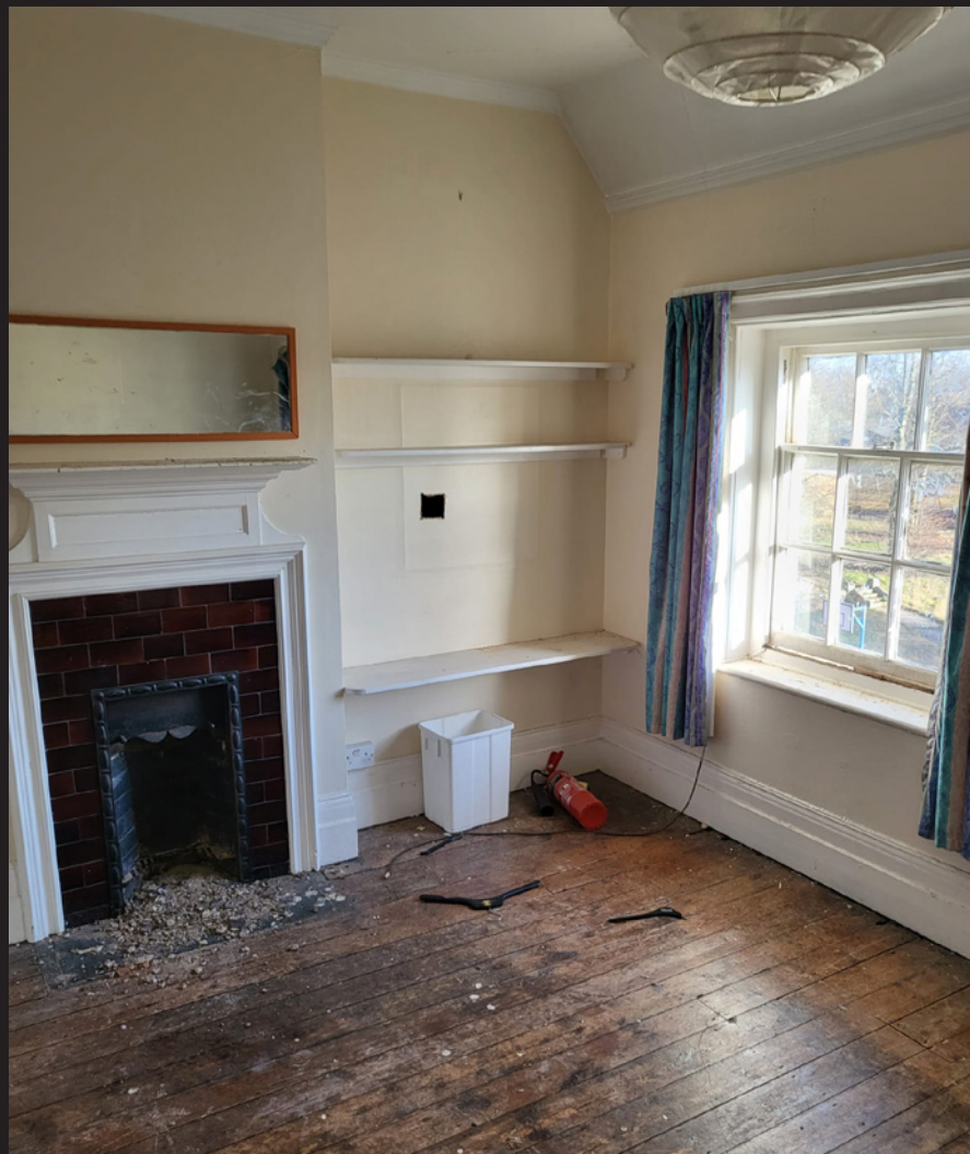
Example of an existing room with fireplace
