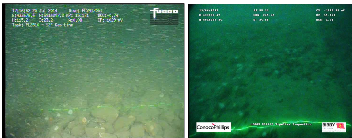
Figure 5-7 ROV footage taken in 2014 (left) and 2016 (right) at the Clipper South pipeline near LOGGS Riser Platform illustrating progressive sand build up amongst the rock since it was deposited in 2012
