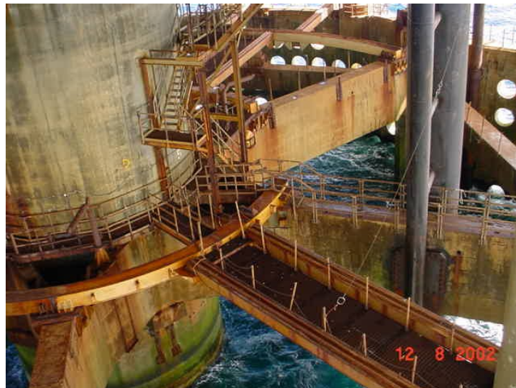
Figure 7.5 Steel works on top of breakwater wall
