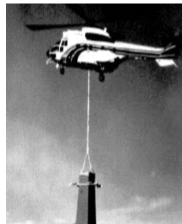
Figure 14.1 Illustration how a helicopter could place the aid to navigation on top of the concrete substructure.
