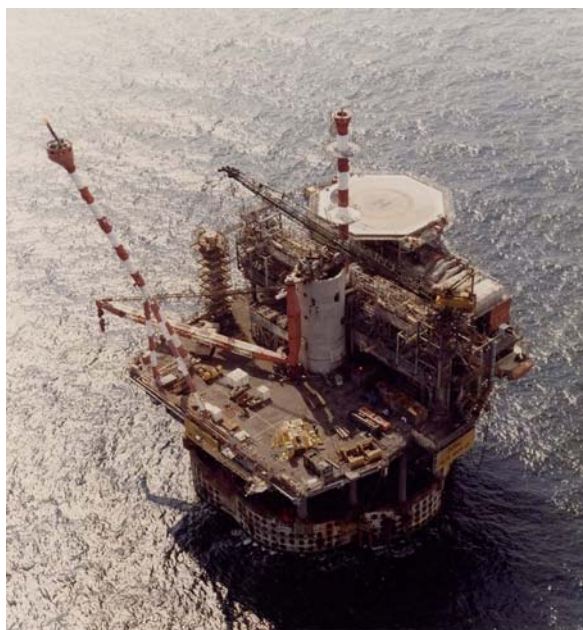
Figure 2.3 MCP-01 before two compression and one treatment modules were installed.
