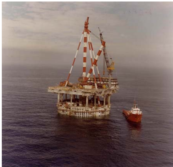
Figure 2.2 MCP-01 during installation of topside facilities.
