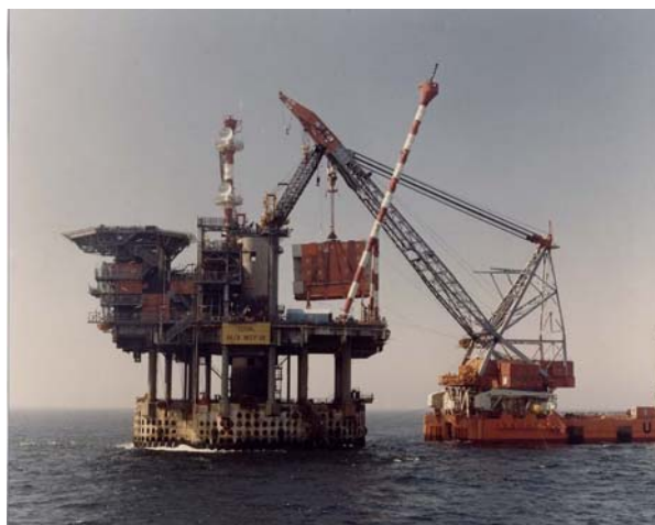
Figure 7.4 Lifting a module on MCP-1
