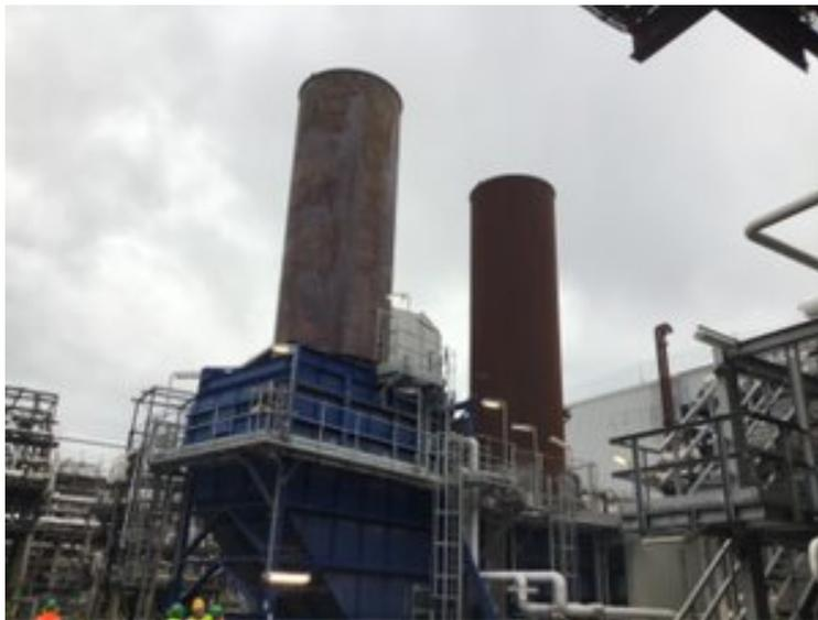
Figure 4-3: SEGAL GT exhaust stacks (Image: Shell)
