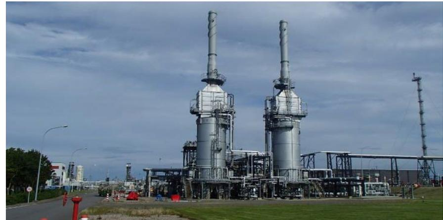
Figure 4-4: FUKA (NSMP) gas fired hot oil furnaces (Image: PX Group)
