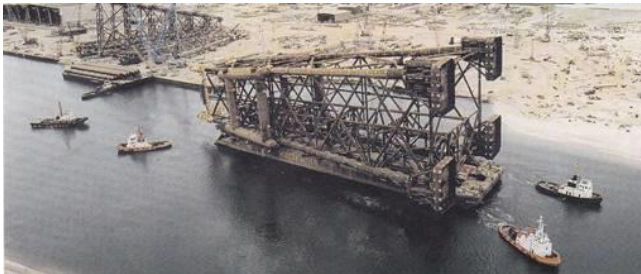
Figure 5.2: Photograph of Saltire A showing the mud mats
