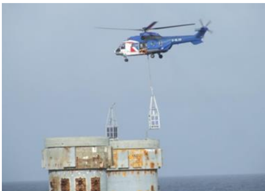
Figure 2-4 AtoN Deployment via Helicopter
