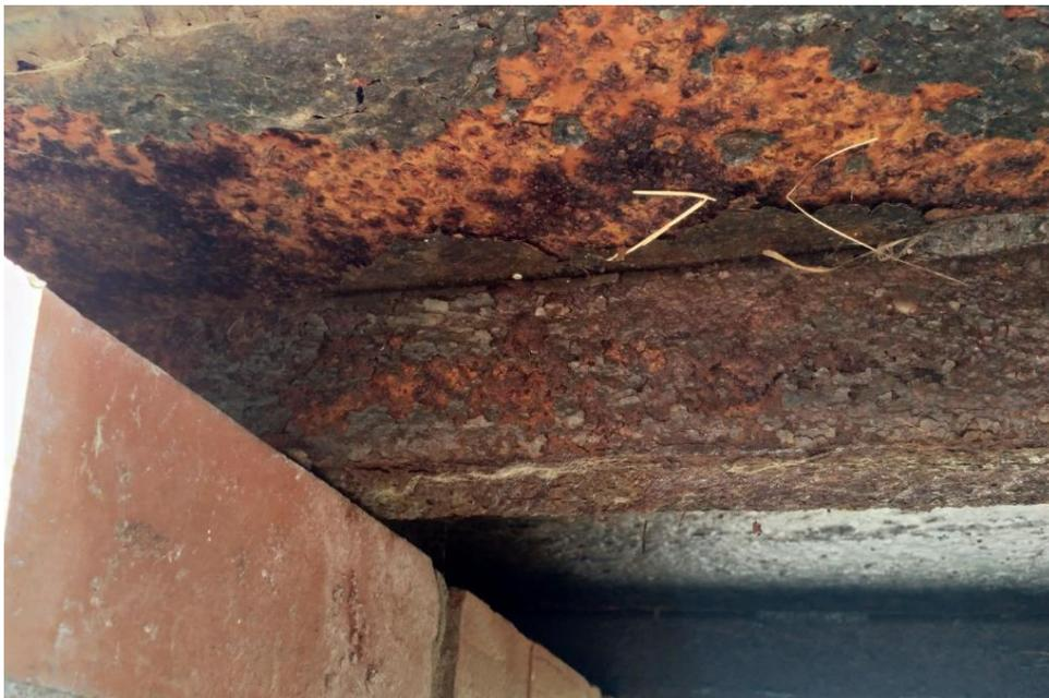
Figure 2: Underside corrosion of secondary tank skin
