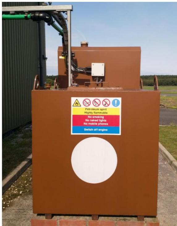
Figure 1: Example of a typical above ground metallic rectangular integrally bunded storage tank
