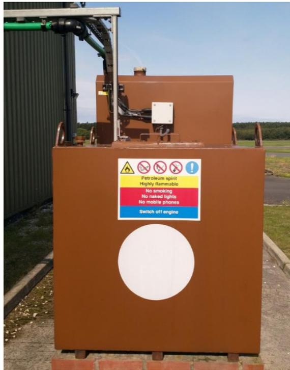
Figure 1: Example of a typical above ground metallic rectangular integrally bundled storage tank
