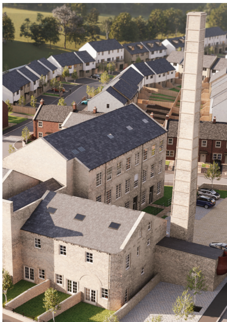
Stonebridge Mills, Leeds, is a key part of the history of the Farnley and Wortley area but has lain unused, in a state of decay for many years. The site, which extends to some 3.6 hectares, includes a complex of traditional industrial buildings, along with former cottages and mill offices, was registered by Croydon office in March 2021. Image: Advent Developments/Rushbond Plc
