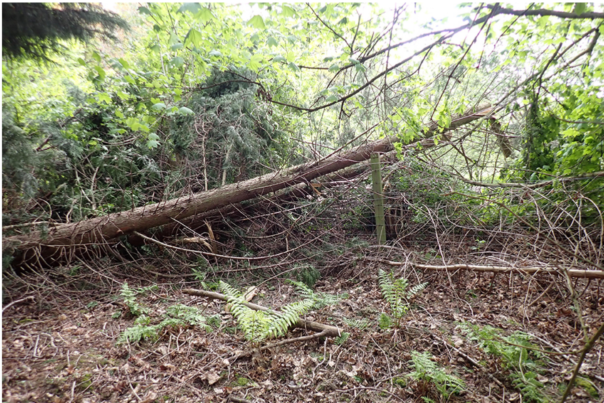
The remains of the fallen tree after the accident, viewed from outside the railway boundary fence, showing the branches which had grown from the fallen trunk and which eventually fell themselves
