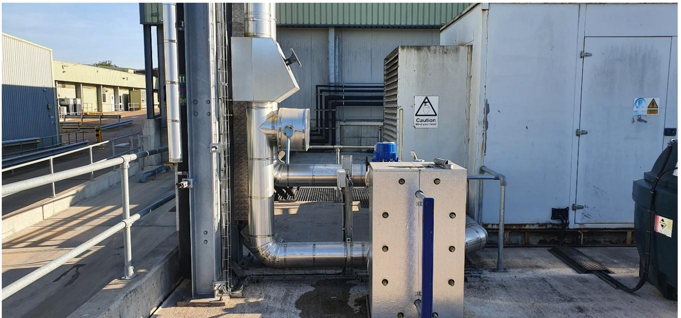
The images provided show the existing chiller units and pipework to which the units designed during the IHRS project would be integrated.
