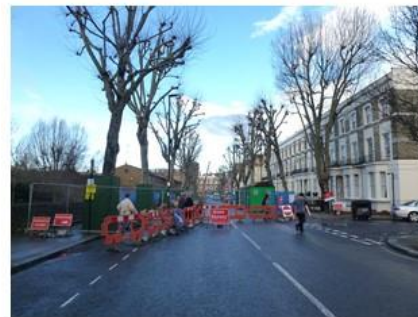
New sewer construction in London
