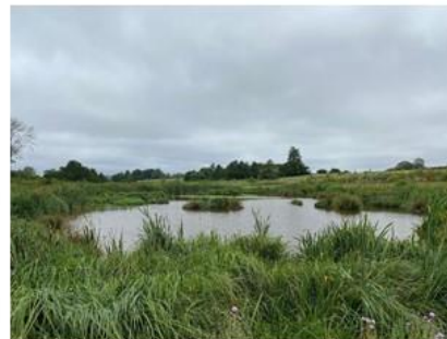
Integrated Constructed Wetlands
