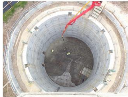
An underground storm storage tank in construction
